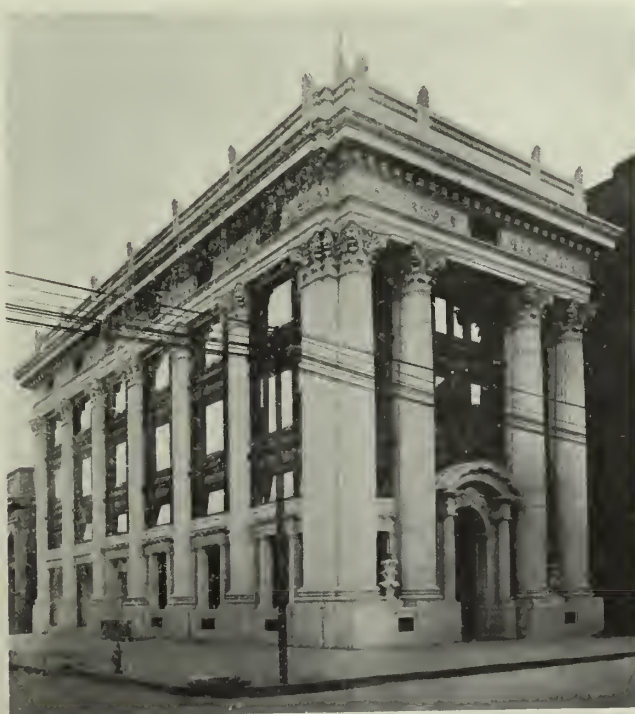
DAYTON DAILY NEWS BUILDING. Exterior treated in Atlantic cream mat terra cotta furnished by Atlantic Terra Cotta Company.
